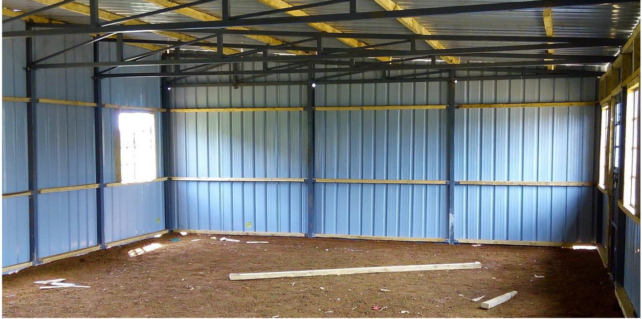
Inside the church building where they are laying the floor today
