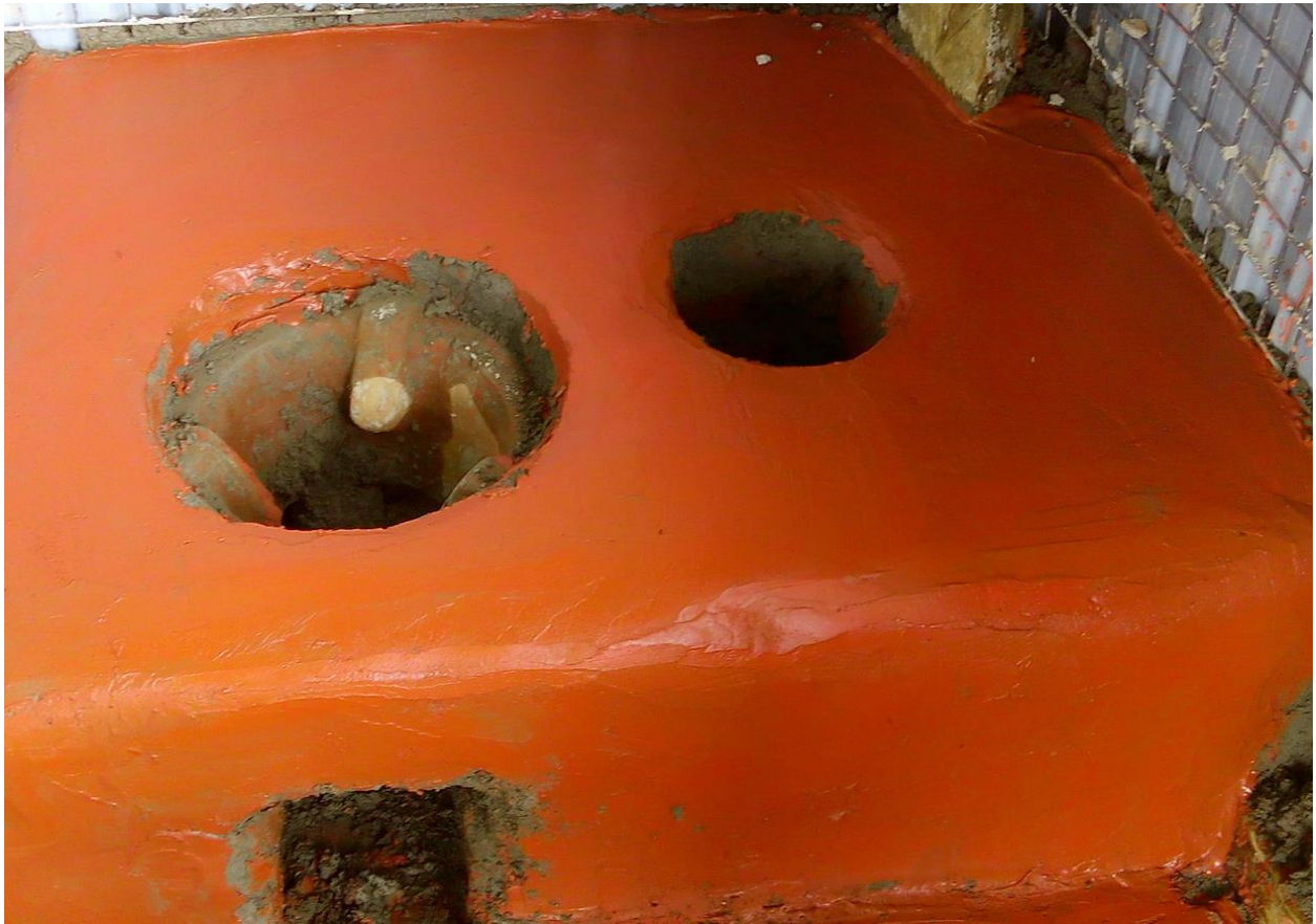
The next day the students made this stove for practice. Note the energy saving liners being used
