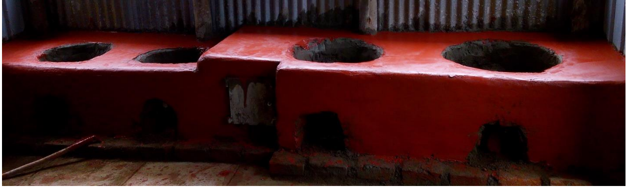
Mr. Kibet from the Ministry of Energy helped teach about making energy saving stoves. This is the four stoves and oven in the middle
